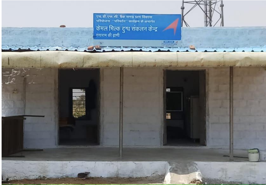
(above) Bulk Milk Chiller of 1,000 litres capacity has been installed in a community centre in Ganga Ram ki Dhani village, Pokaran camel milk cluster
